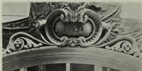
DETAIL BY KETCHAM TERRA COTTA WORKS. Ben R. Stevens, Architect.
